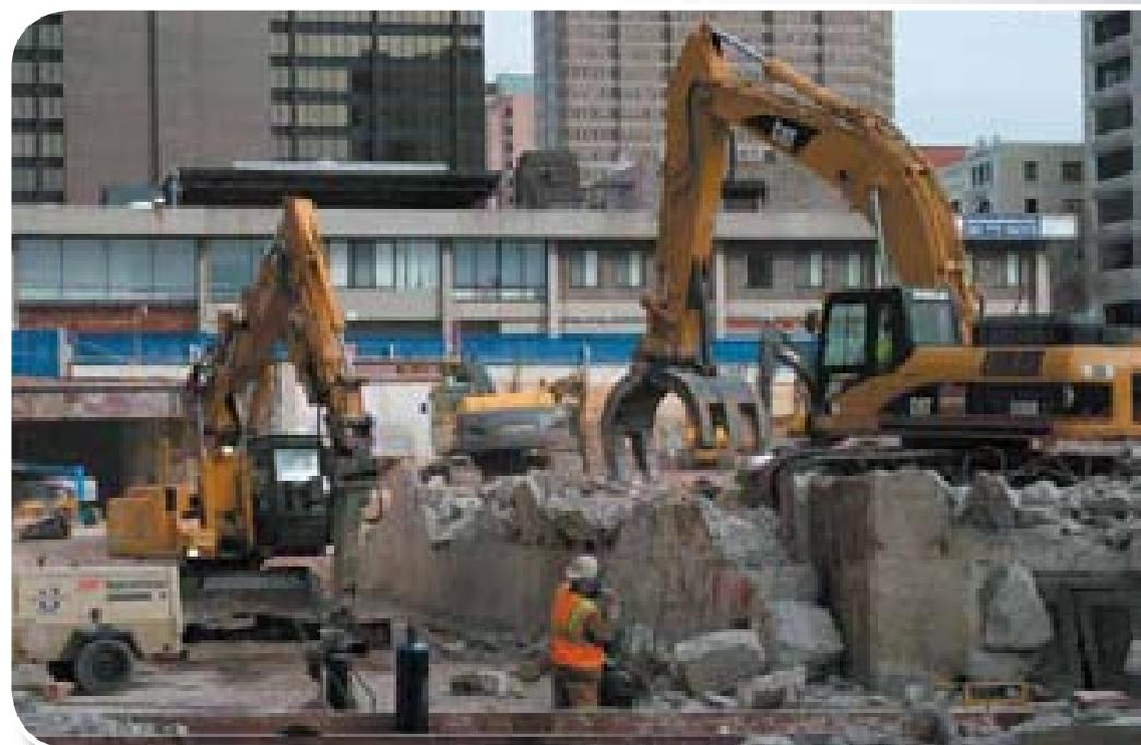
*Worker wearing respirator observes demolition of New Haven truck tunnel by Laydon Industries' CAT 330D, John Deere 210C and Volvo EC360B excavators.*
