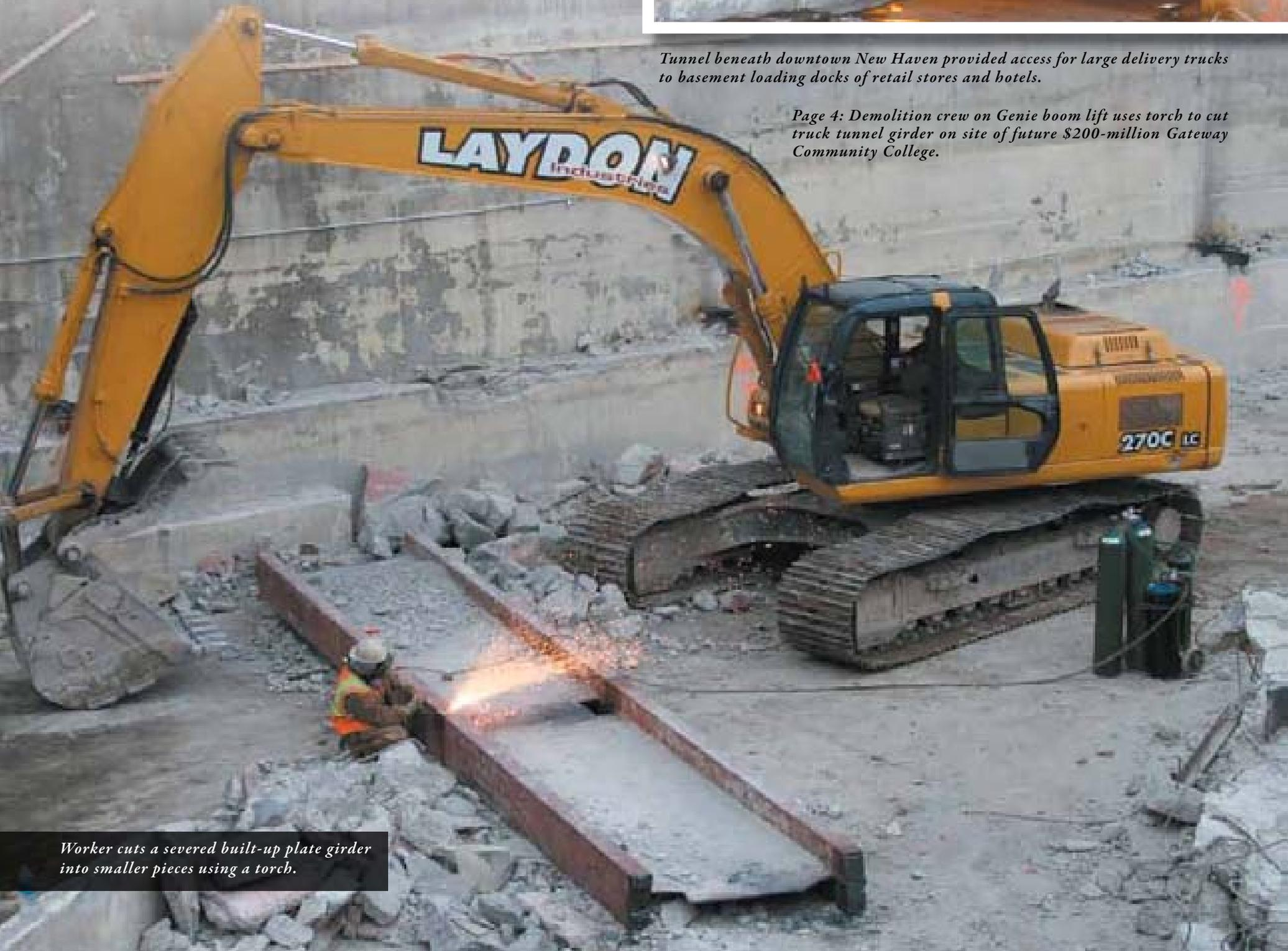
*Worker cuts a severed built-up plate girder into smaller pieces using a torch.*
